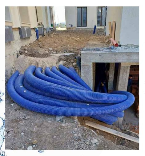
For the project, 18 Microflex® DUO pre-insulated flexible hoses of different lengths (the longest being 95 m) were used for a total of more than 900 metres (about 10 football fields lined up one after the other)!
