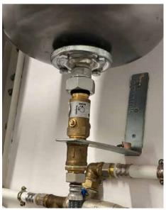
To compensate for variations in the volume of the heat transfer fluid in the heating circuit, the ACS/AFE expansion vessel has been installed, which prevents increased pressure in the system from damaging pipes and components.
